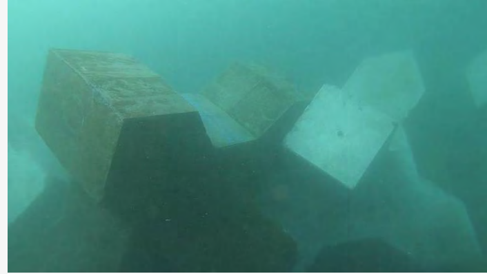
Diver-assisted inspections and underwater video verification
