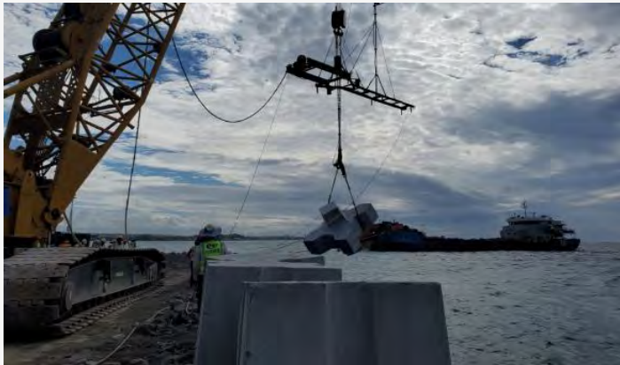
Placement of primary armour units (Xbloc system)
