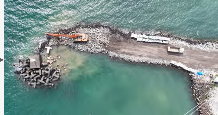
Retain and build upon the existing core. New breakwater alignment is slightly offset, with a widened footprint extending into greenfield areas.
