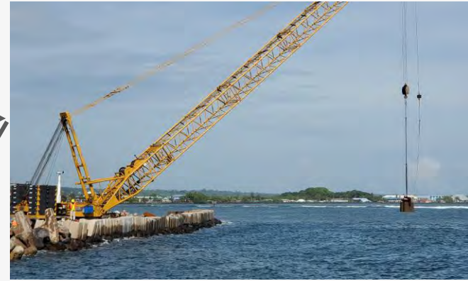
Placement of antifer units
