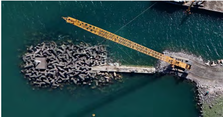
Removal of existing Dolosse armour units & Concrete Crown Wall.
