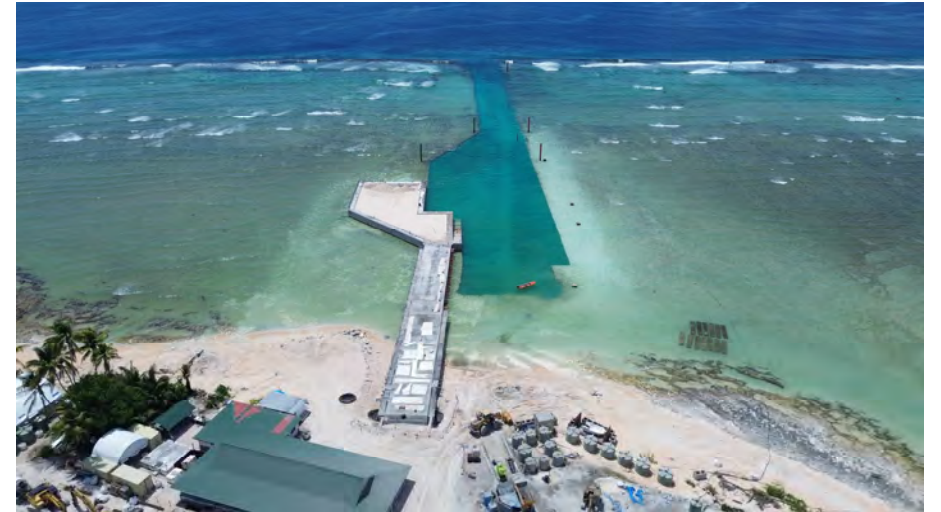
Nui Wharf, Tuvalu Source: Hall Contracting
