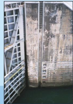
Lock wall deterioration, Chickamauga
