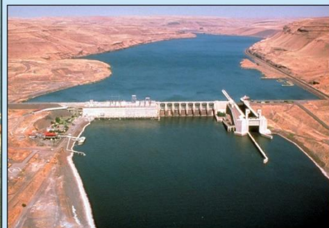
Tows on Columbia/Snake system in Pacific Northwest use unique locks with lifts over 100 feet.
