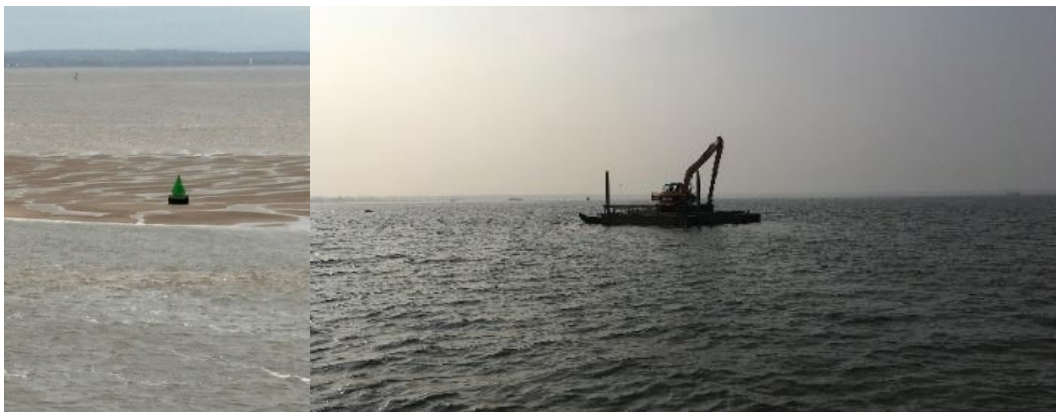
Photo 1 and 2. Climate-related changes including more frequent storms can affect sediment dynamics, requiring additional surveying and impacting dredging requirements. Photo 1 on left shows channel edge marker buoy, in its charted position but aground after a storm in the Mersey, UK, April 2024. (Photos: Peel Ports Group, UK, and Jan Brooke, PIANC)
