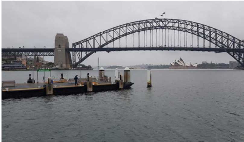
FIGURE 1. IN THE FOREGROUND, A FERRY COMMUTER FLOATING PONTOON LOCATED AT MCMAHONS POINT IN SYDNEY HARBOUR, AUSTRALIA.
