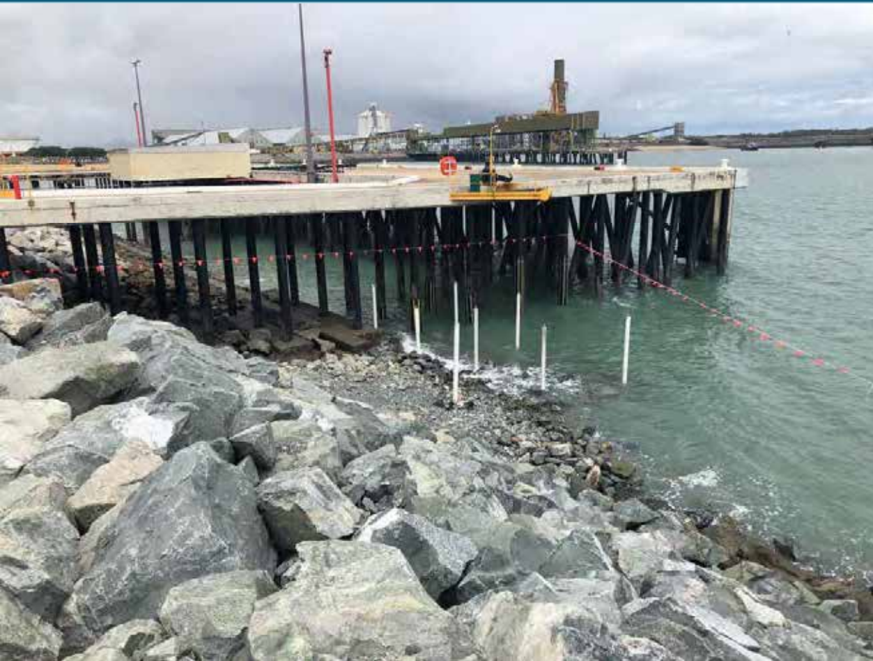
Stability berm completed and monitoring markers installed
